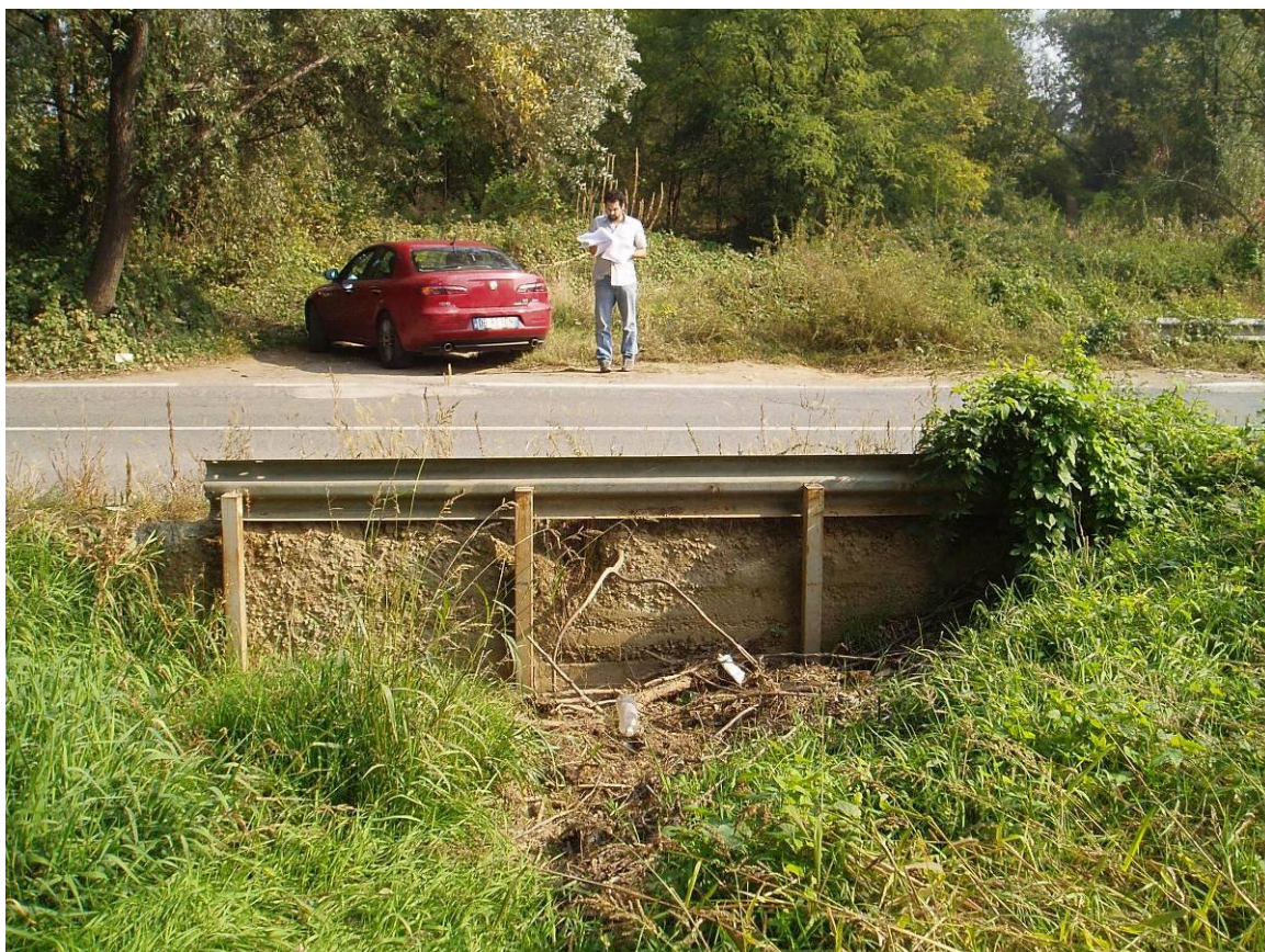
001ANSEAG001 – Vista da monte (foto 923-PA100025)
